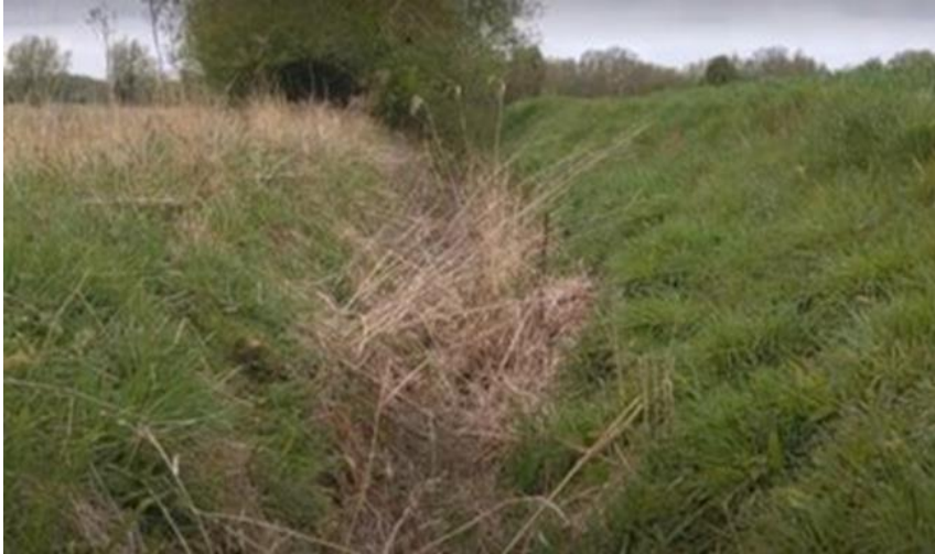
Photo 1 Existing ditch along northern boundary of area Works No. 39
